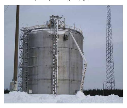
Fig. 3. Large LPG Storage vessel with AE ISHM System "Recourse-M" 1993.
