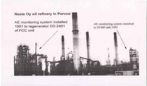
Fig 2 AE monitoring Systems at Neste Oy Refinery
